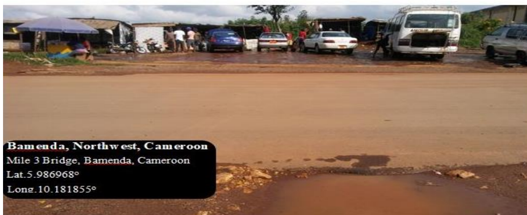
Figure 6: Absence of pedestrian paths, road signs/markings and parking lots along Mile 3 Bridge in Bamenda II
